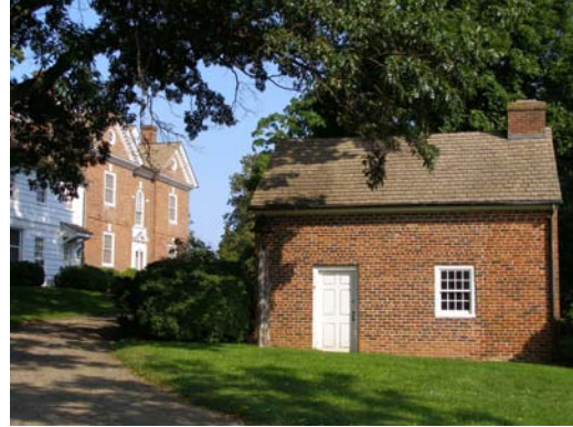
Colonial Kitchen, after restoration.
