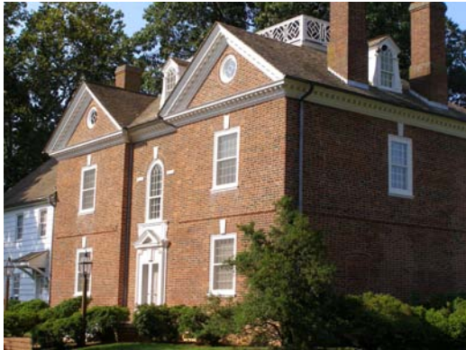
Mount Harmon Manor House, after restoration.
