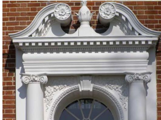
Manor House front entrance, after restoration.
