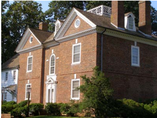
Mount Harmon Manor House, after restoration.
